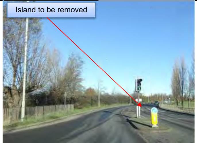
8.4.6.4. – View on junction
