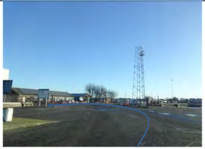
8.4.1.2. – View prior to junction
