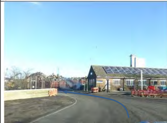
8.4.1.3. – View at crossing
